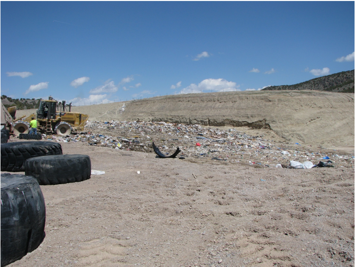
Looking at the working face of the MSW cell
